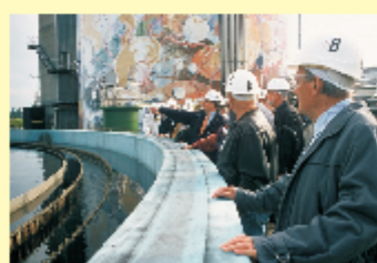
Honeywell invested in the cover for the settling basin of the water treatment plant to reduce odour emissions.
