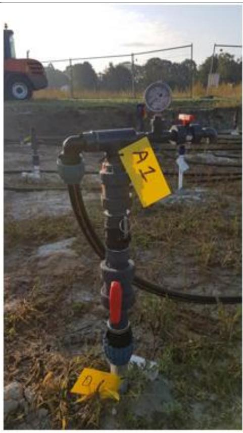
Detail injection well manifold
