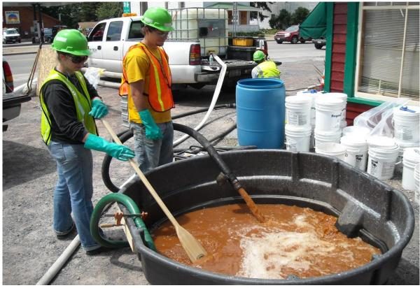
Figure 2.5- Mixing reagents before injection
