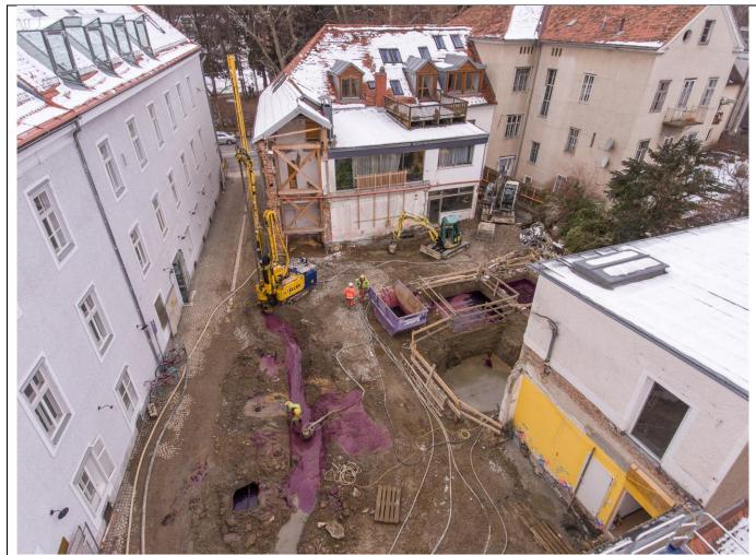
A picture of the site. Works are conducted below former washing machines. Backflow deeply covered purple by  $\mathsf{KMnO}_4$
