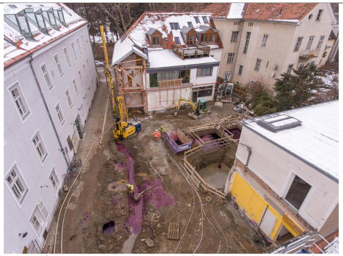
A picture of the site. Works are conducted below former washing machines. Backflow deeply covered purple by KMnO<sub>4</sub>
