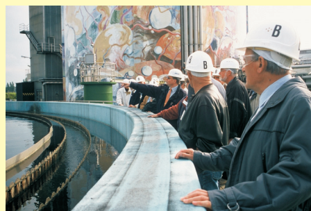
Honeywell invested in the cover for the settling basin of the water treatment plant to reduce odour emissions.
