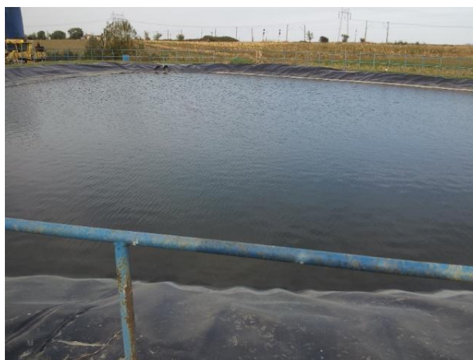
Figure 35: Lagoon for treated leachate water at Landfill in Romania
