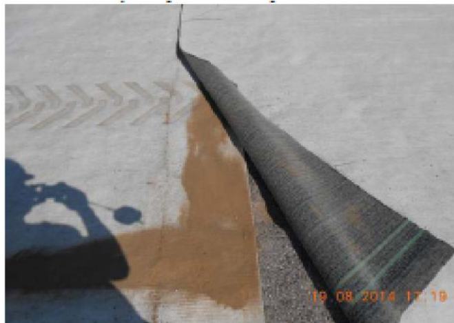
Figure 48: Geosynthetic clay liners
