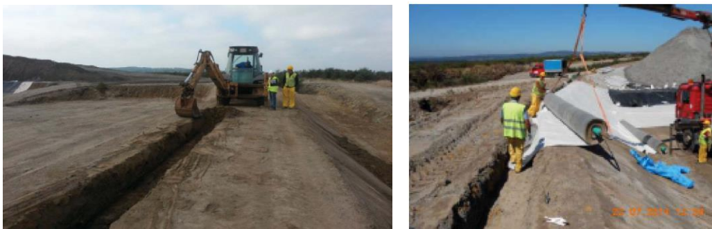
Figure 44: Trenches in coronation slope
