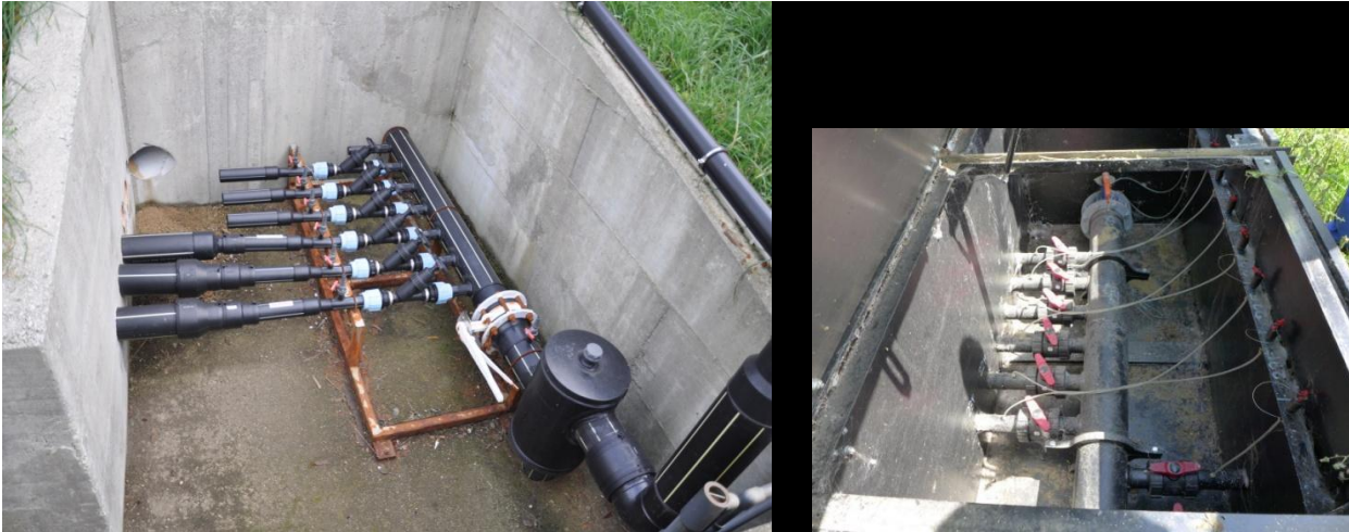
Figure 25: Landfill gas piping
