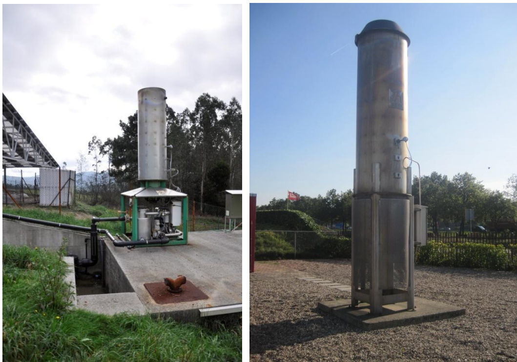
Figure 23: Landfill gas flares examples
