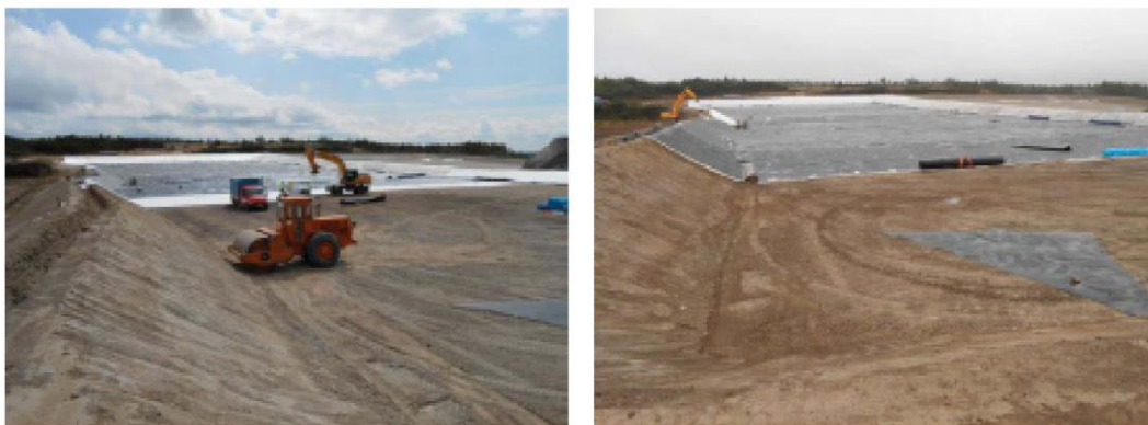
Figure 39: Bottom and slope of the cell
