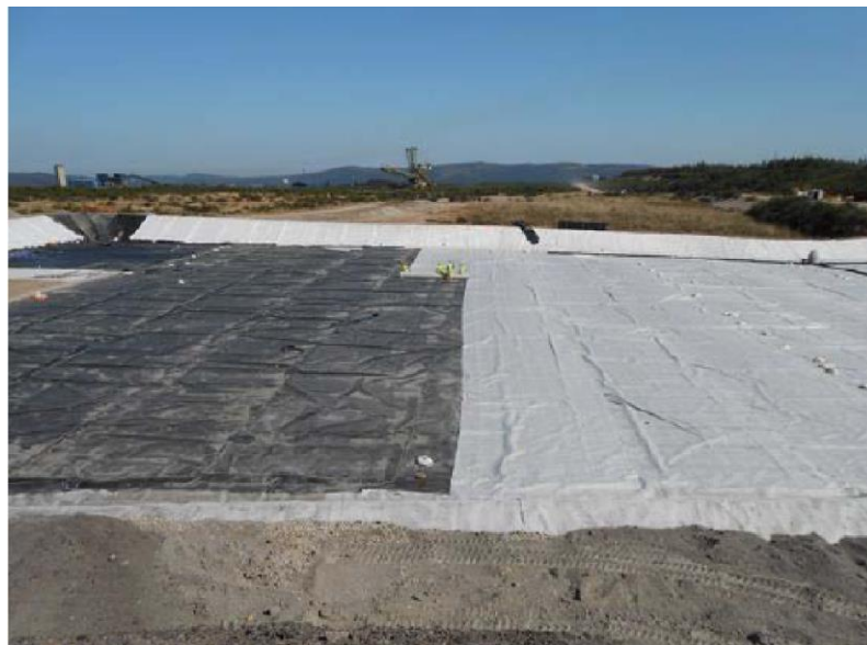
Figure 50: Geotextile protection
