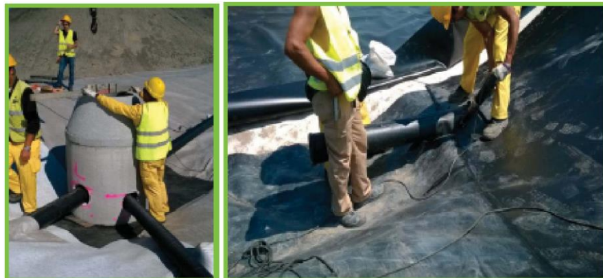
Figure 45: Anchoring systems
