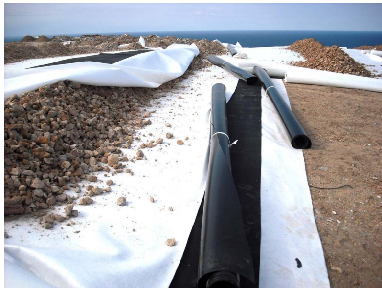
Figure 52: Geotextile filter
