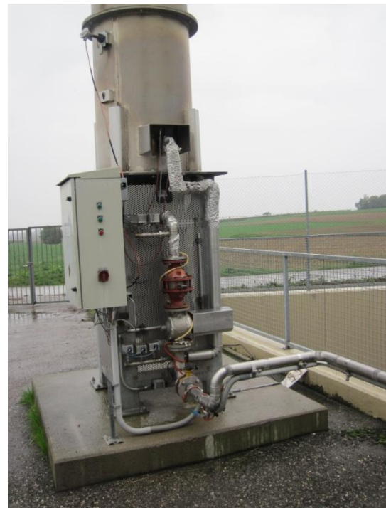
Figure 22: Landfill gas flare
