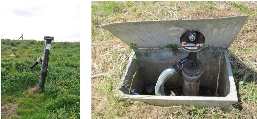
Figure 19: Landfill gas collection boreholes
