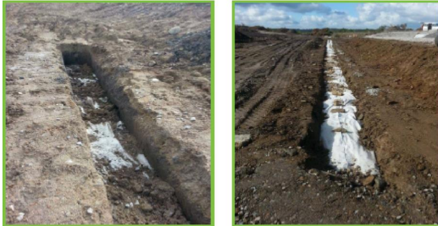
Figure 40: Groundwater collection network
