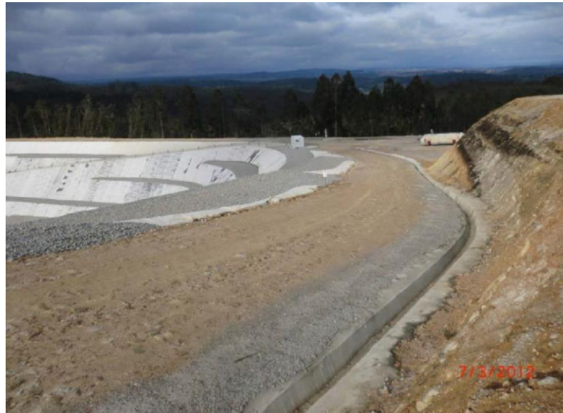
Figure 58: Ditch perimeter of rainwater
