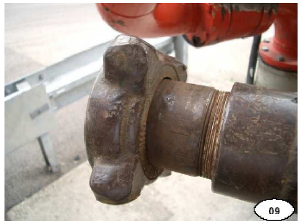
Examples of worn threaded coupling : road-tanker fitting and threaded ring
