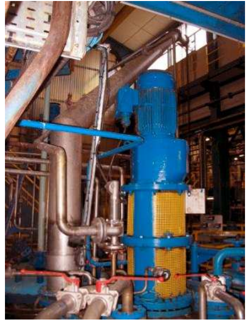
Upper part of the reactor: mixer and burst disk discharge line
