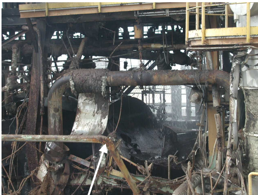
Fig. 4 – tank D 528/1 : 2 nd explosion
