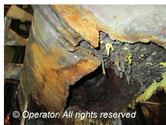
Sulphur leak from the heat exchanger
