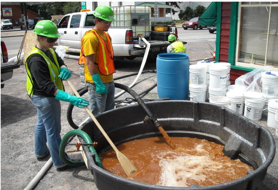
Figure 2.5- Mixing reagents before injection
