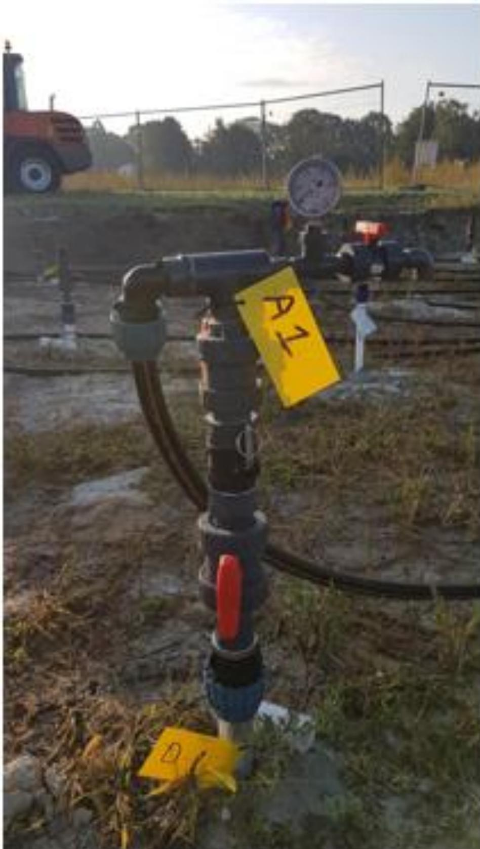
Detail injection well manifold
