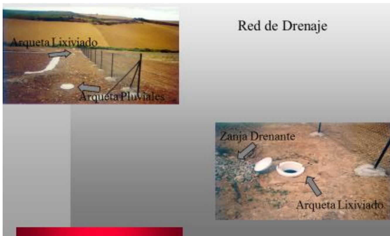
Figure 2 - Installation of drainage ditch and water collection pit
