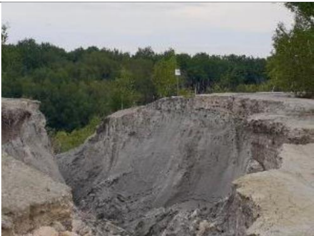
Figure 2 - Erosion of tailings on the Abbaretz mine
